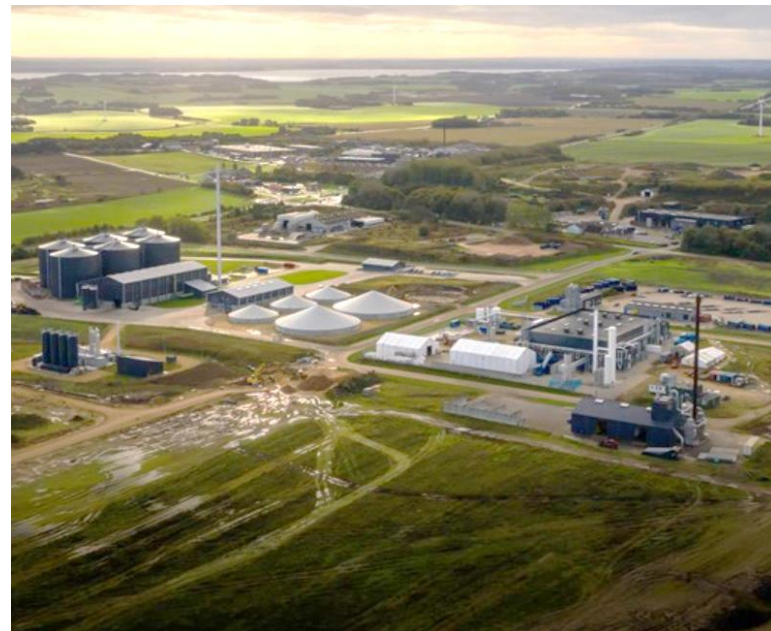
Illustration: Biogas and coming PtX plant: GreenLab Skive
