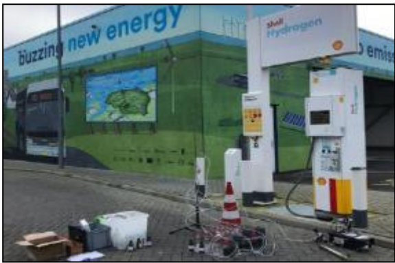
Commissioning hydrogen fuelling stations
