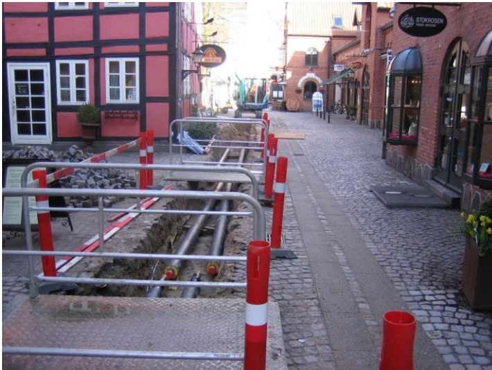
Pipes dug down in the street
