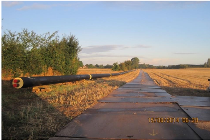
Pipes ready to be dug down in open field
